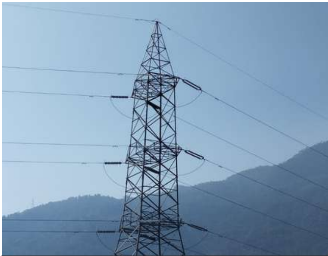
Successful Hotline Stringing for Kusma-Lower Modi-New Modi 132 kV Transmission Line
