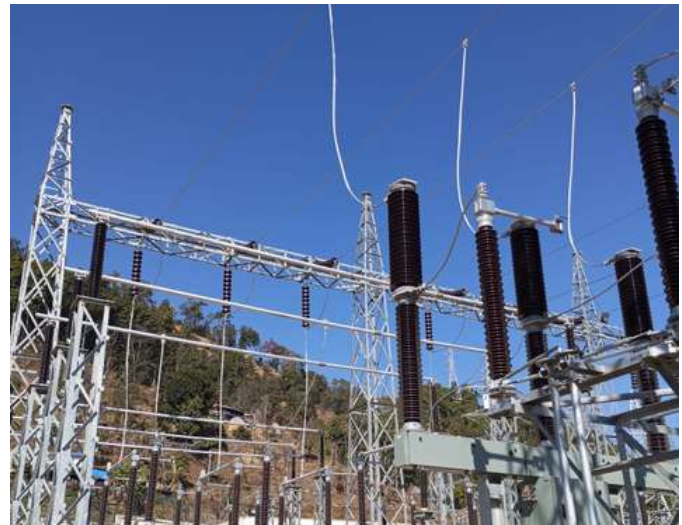
Bay Expansion Milestone for Kusma-Lower Modi-New Modi 132 kV Transmission Line
