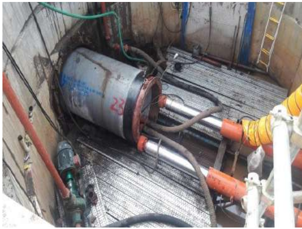
Figure 1: Pipe Jacking operation
