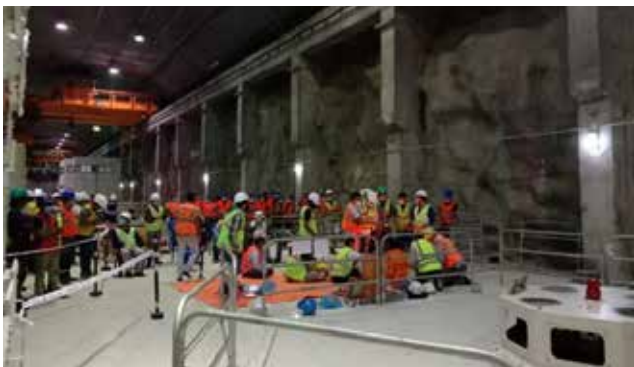
Upper TamaKosi post commissioning
