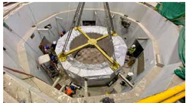
Middle Bhotekosi stator lowering
